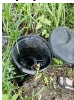
Installed the submersible pump, inside a black plastic bin for protection
