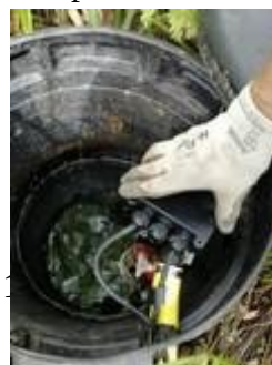
Installed the submersible pump, inside a black plastic bin for protection
