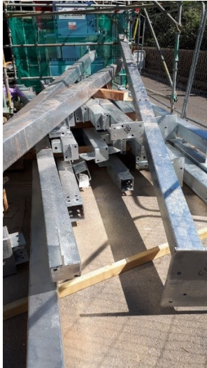
Steel frame delivery for the green walls to the front of buildings H&L Large Meccano set
