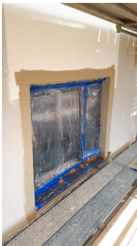
Decoration and render panels prior to fitting brise Soleil
